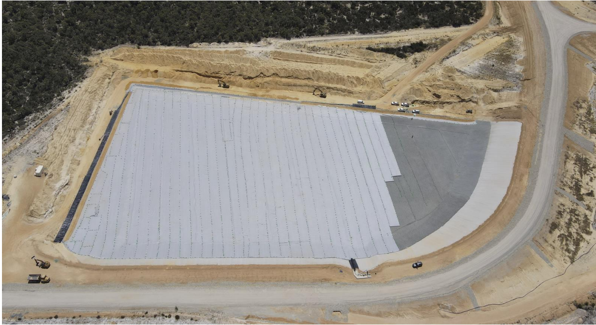
Figure 1: Cell 1 completion imminent
