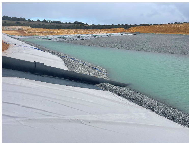
Image 2: Cell 1 - Final layer installation
