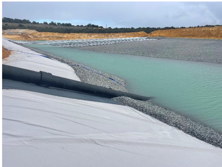
Image 2: Cell 1 - Final layer installation
