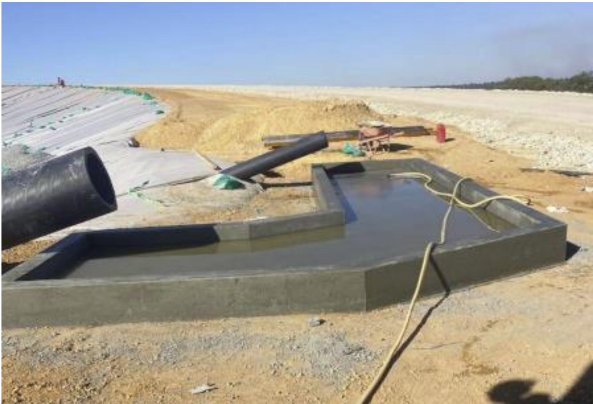
Image 2: Leachate pumping station concrete pad
