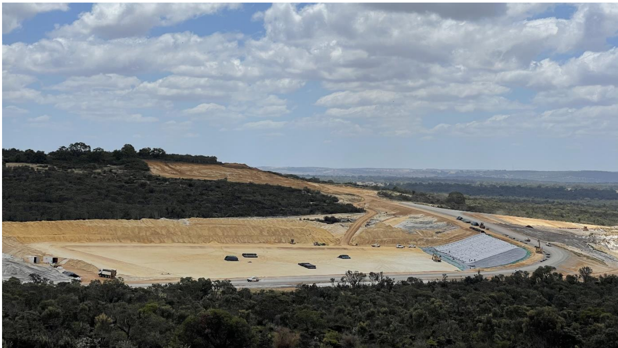
Figure 1: Bioreactor Cell 1 Liner Installation
