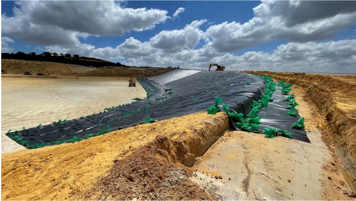
Figure 2: HDPE Liner - 1st layer
