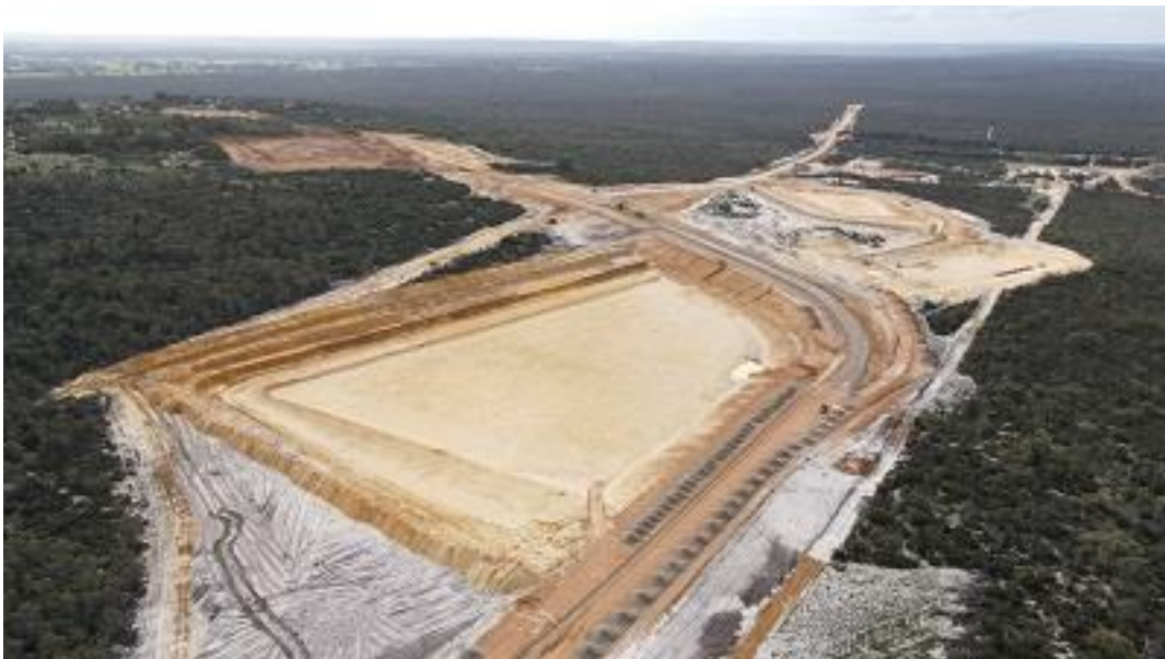
Image 2: Cell1 and ring road construction
