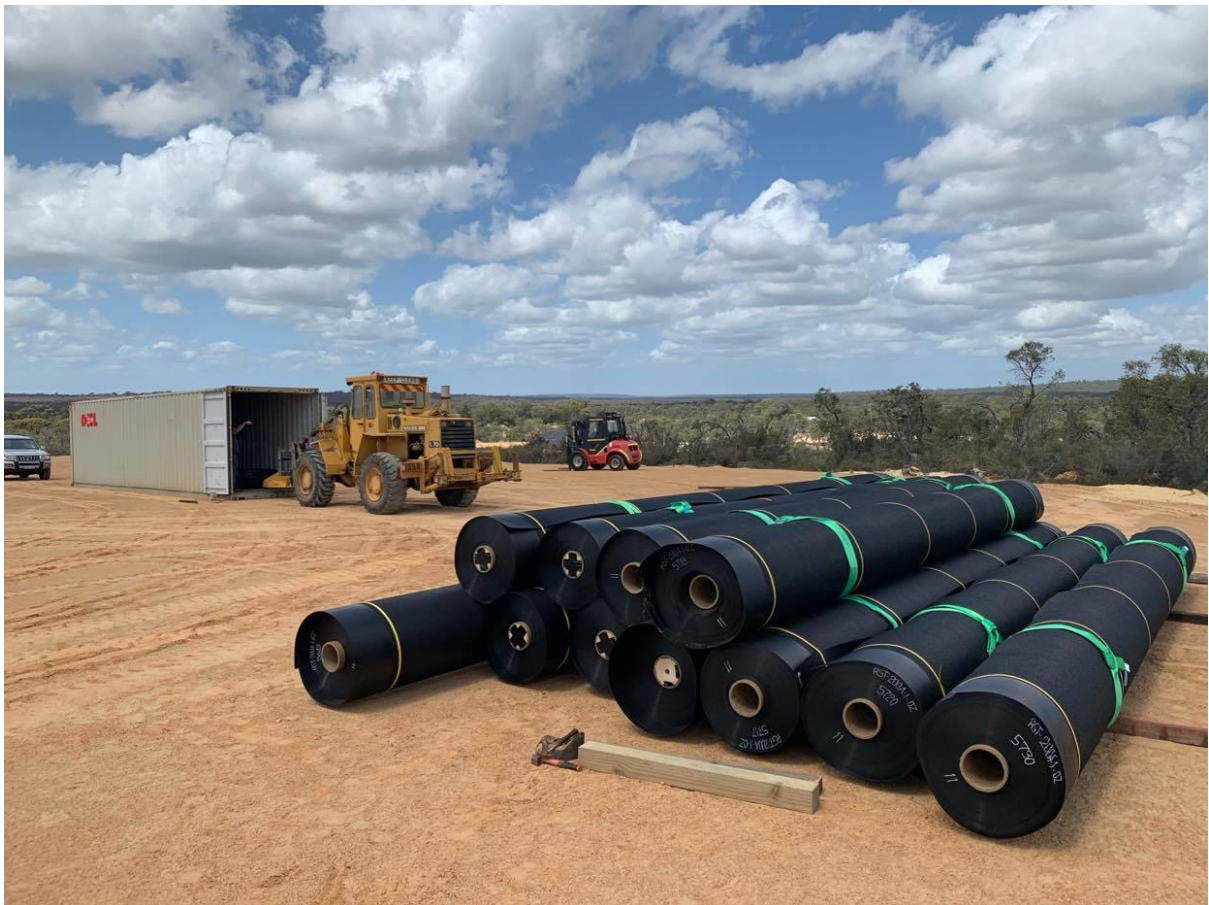
Figure 3: HDPE Liners to be installed at Gingin
