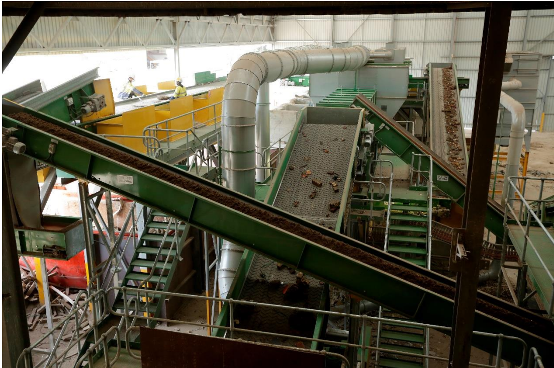
Figure 3: C&I Recycling Plant
