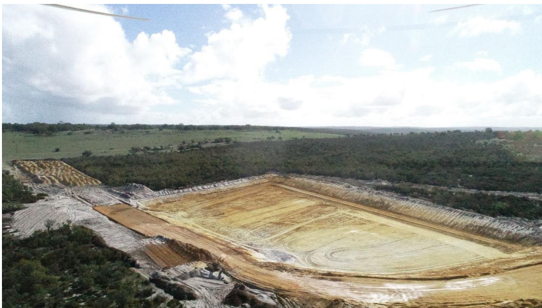
Picture 1: Cell 1 Earthworks
