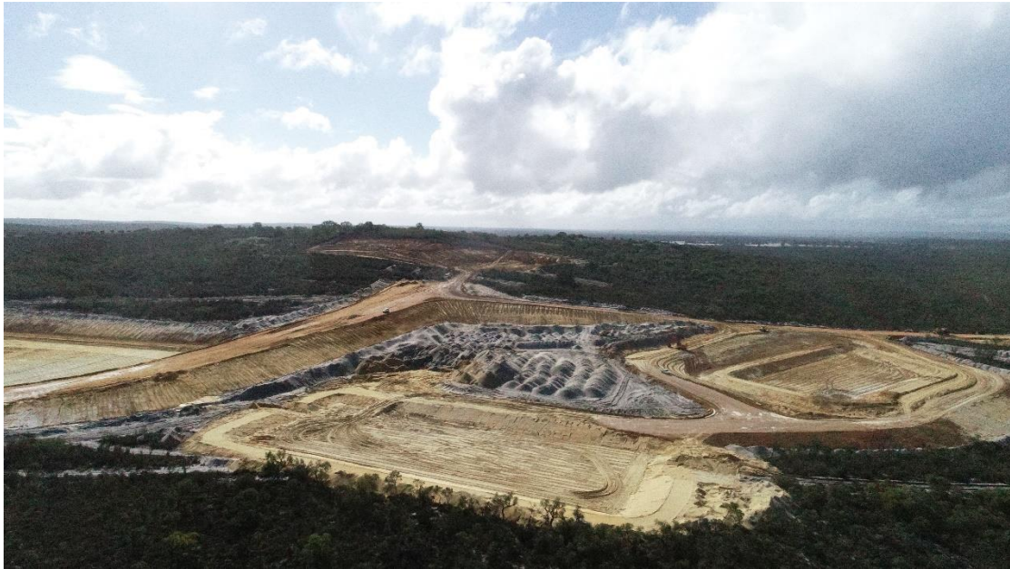
Picture 2: Leachate & Settlement Pond Earthworks
